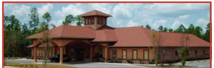
Our recently completed 10,600 sq. ft. office in Milton, FL
